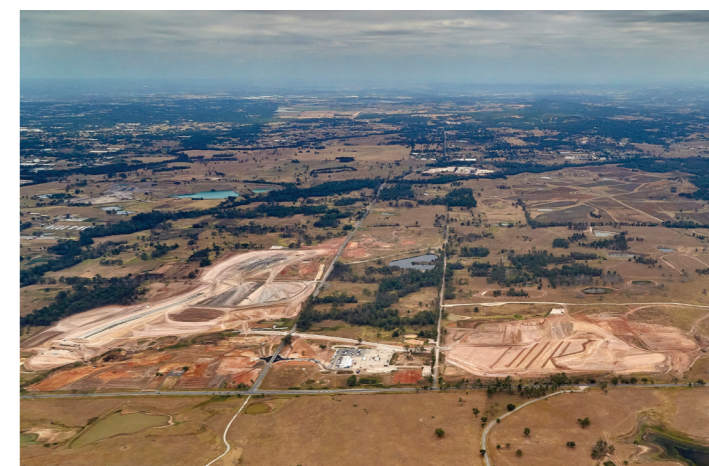
Early earthworks, March 2019
